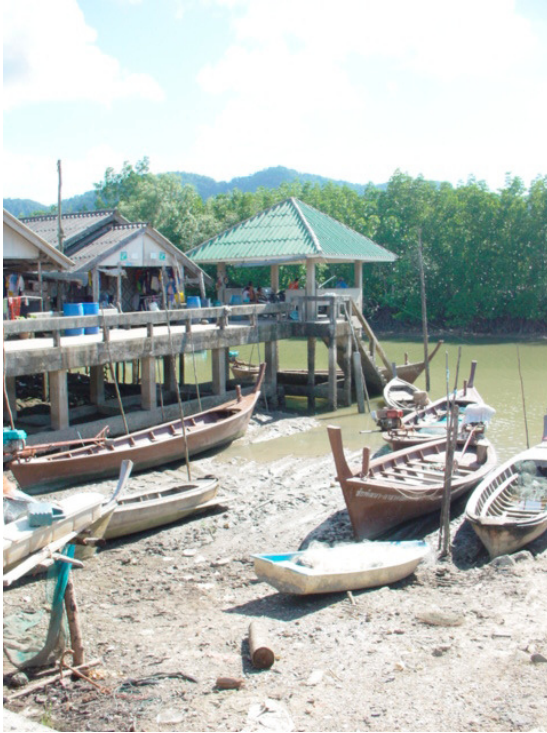
Construction of Stopping Point
