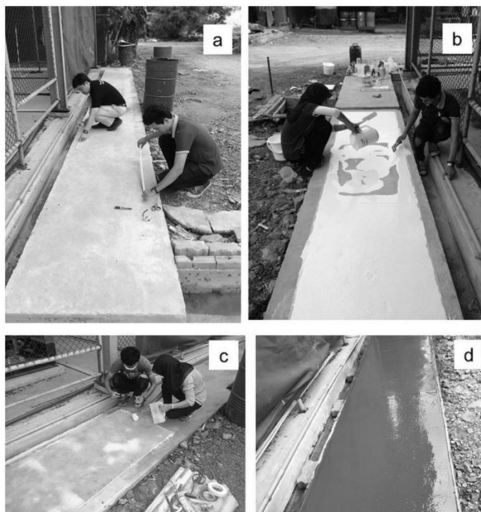
Fig. 3. Large-scale rubber flooring sheet prepared from the optimized condition (a) surface preparation (b) applying optimized condition on cement (c) after curing under sunlight for 6 h and (d) surface coating.
