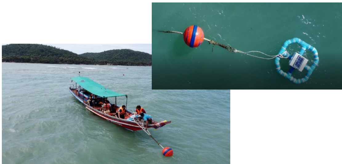
Fig. 28. Installation of pontoon.
