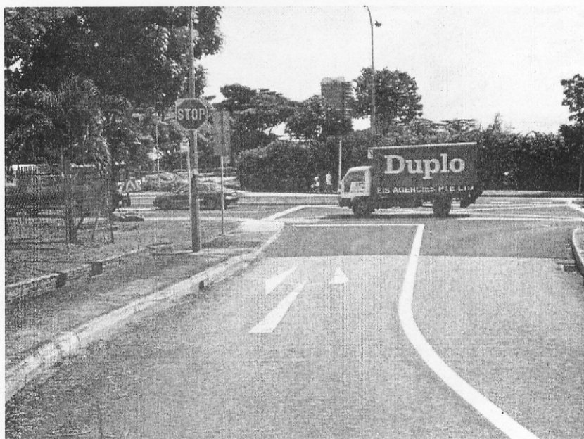
Improper location of "STOP" sign (4).
