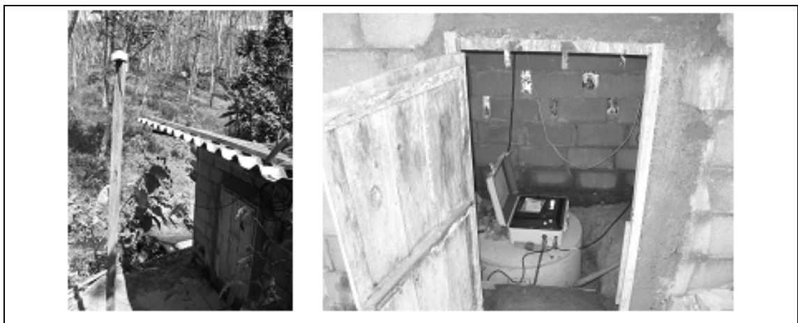
Figure 2.7. Left : Station is located near the waterside. There is a small concrete shelter containing a concrete tube and the Orion portable seismograph and a GPS antenna in front. Right : Concrete shelter where the Orion portable seismograph is protected in the concrete tube.
