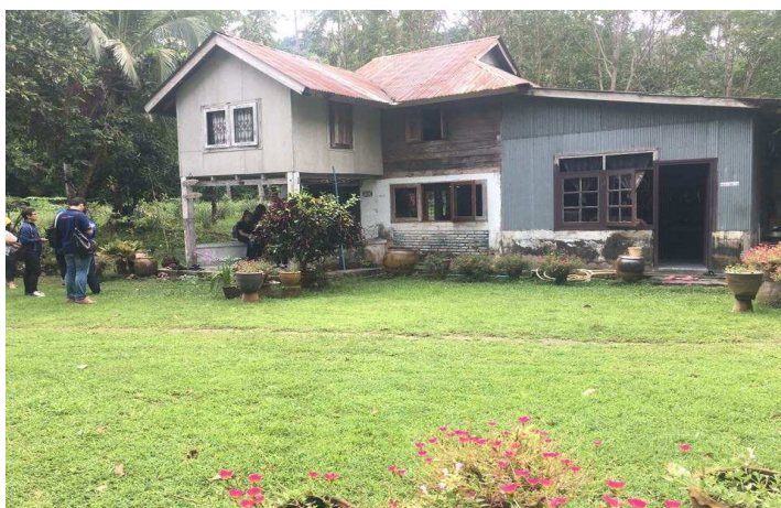
Figure 5.3 Baan Roi Pee /Ancient House before renovation
