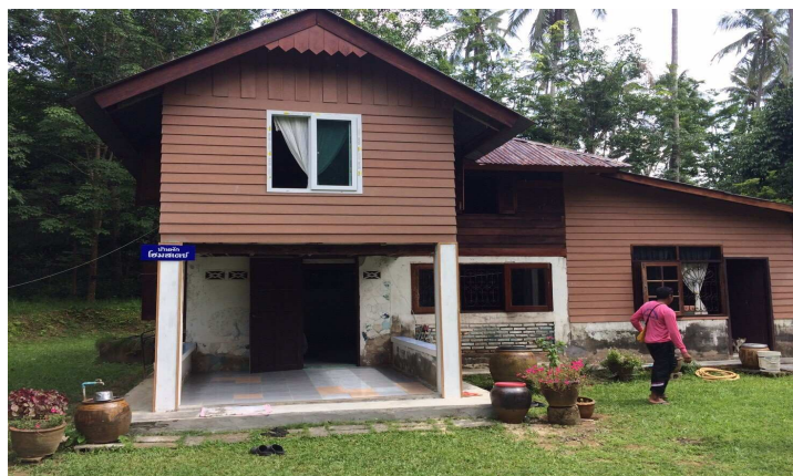
Figure 5.4 Baan Roi Pee /Ancient House after renovation
