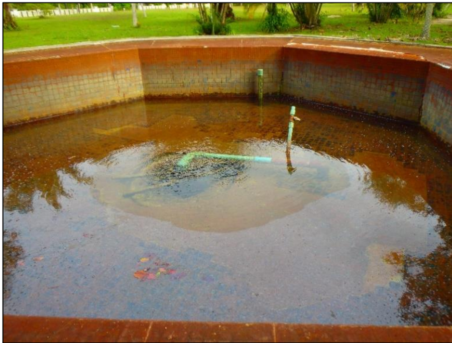
Figure 3.13 One main hot spring spot in PG3 connects with a pipe that flows thermal water to a tourist pool.
