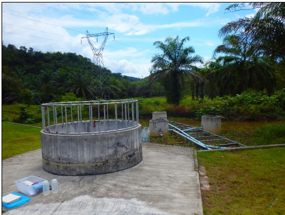
Figure 3.11 Hot springs in PG2 discharge into a canal and some overflow into the mainland.
