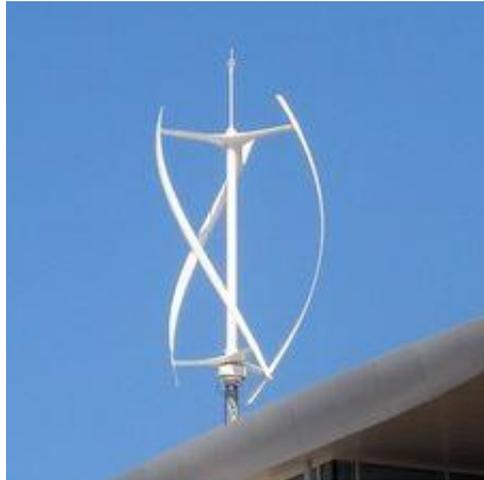
**Figure 2.6** A Vertical axis wind turbine for electrical generation
