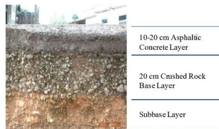
Fig. 1. Material Layers of Pavement Structure.
