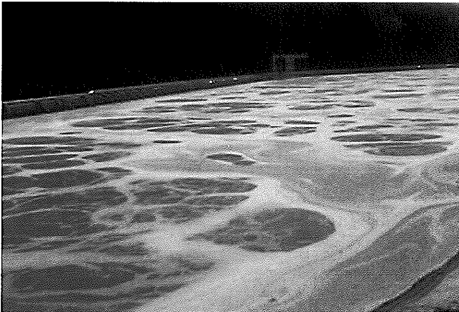
Figure 20. Foaming and bulking in aeration pond of rubber latex processing plant on March 2008.
