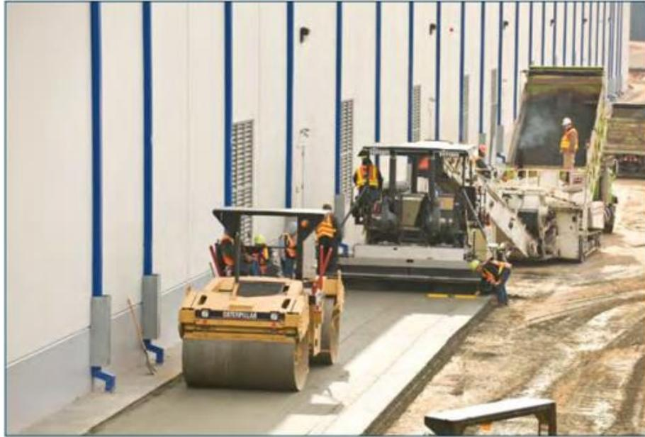
Figure 3. The placement and compaction of RCCP
