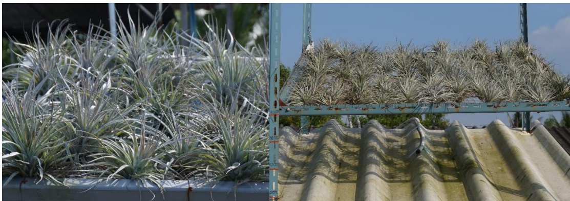
Figure 1.9 Tillandsia recurvifolia Hooker "Tillandsia Cotton Candy" air plant green roofs (Sloping on roof structure)
