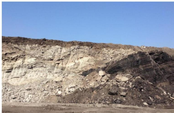
Fig. 4. Cut slope of C1 West wall section fifth in Mae Moh coal mine, Lampang, Thailand.
