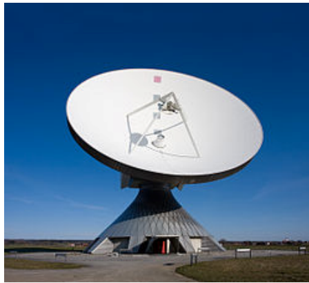
Fig. 2.9 A parabolic satellite communications antenna ( http://en.wikipedia.org/wiki/Parabolic_antenna )
