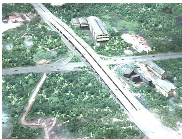
Figure 2.4 Flyover intersection type
