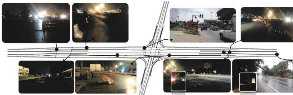
Figure 6. Traffic signs and road marking issues
