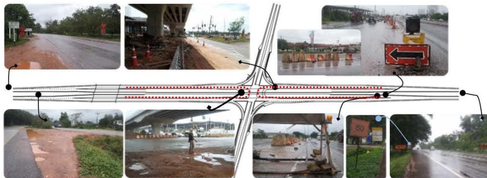
Figure 5 Issues: Traffic management
