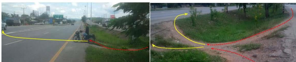
Fig. 6. An illegal movement at the drainage ditches on the median of the road.
