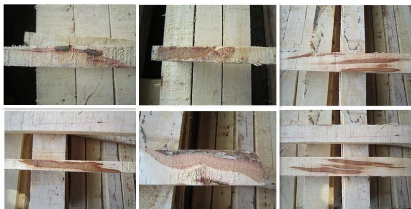
Fig. 4.6 Defects with irregular shape(s)
