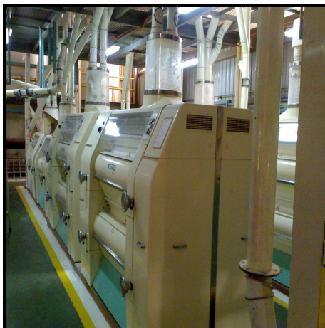
Figure 1.9 Break roller mill for wheat grinding
