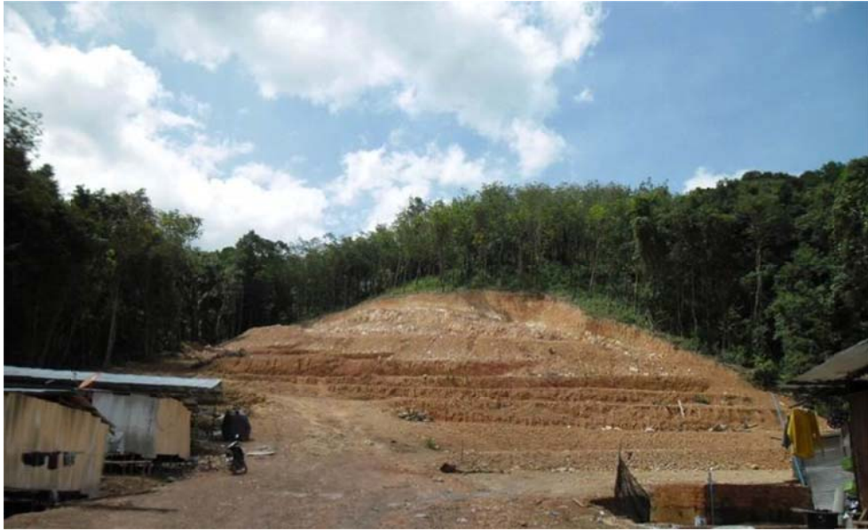
Figure 3.2 Location with mainly sandstone. View to North.
