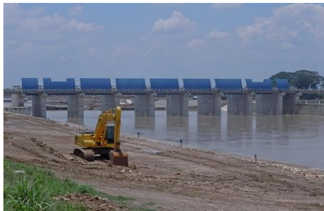
Figure 4.4 New Dam in Bojonegoro Regency Source: Researcher's Document (2 nd November 2011)
