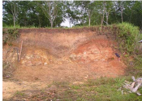
Fig. 3: Site Vibhavadi V1. Almost vertical face at a former sand pit. Photo to direction 160 (SSE). Scale (left side) 2 m.
