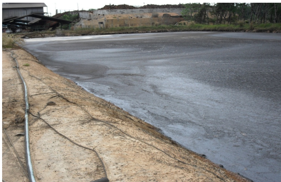
Figure 4.1 The first anaerobic pond.
