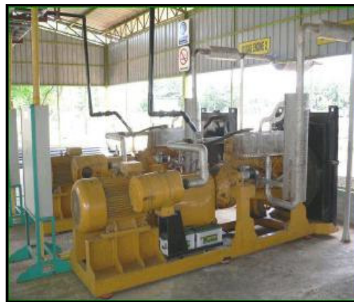
Figure 6. A modified diesel engine operated by biogas
