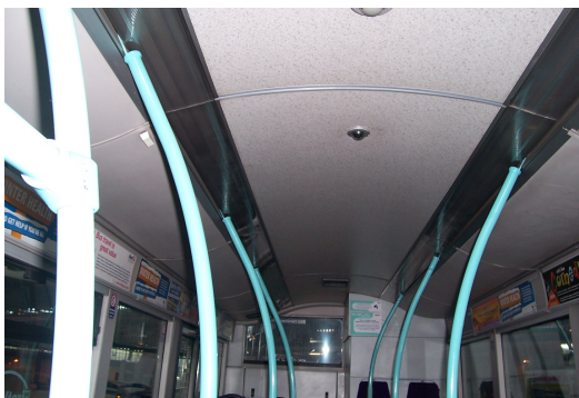
Radio and CCTV camera in roof
