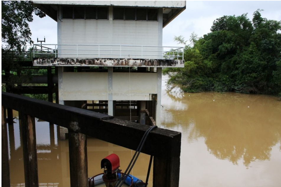
Figure 3.2 Sampling site at a pumping station, Hat Yai Provincial Waterworks Authority
